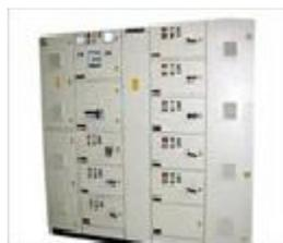
UPS: We used 2 numbers of Emerson 40KVA UPS in parallel with half an hour of battery backup. The ideal situation would be to have UPS working parallel in N+1 mode that means if for example you have a 70KVA load you should use two numbers of forty KVA
